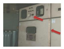
Gambar 5: Medium Voltage Distribution Panel (MVDP)
